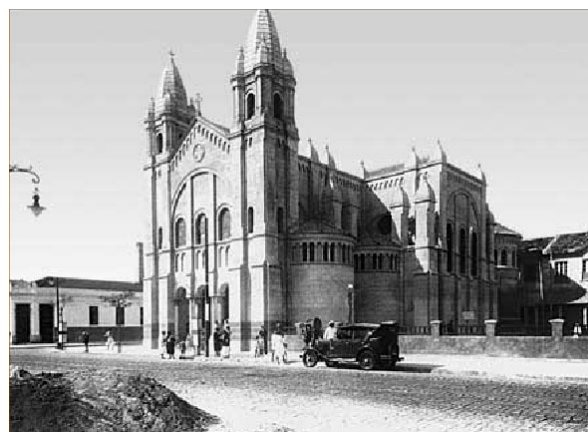
Image 03 – Church of Our Lady of Peace / Ipanema (1921), under construction, still without the tower,
