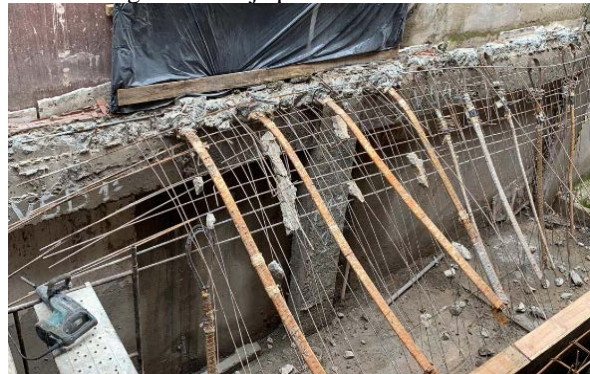
Figura 24: Laje protendida demolida
