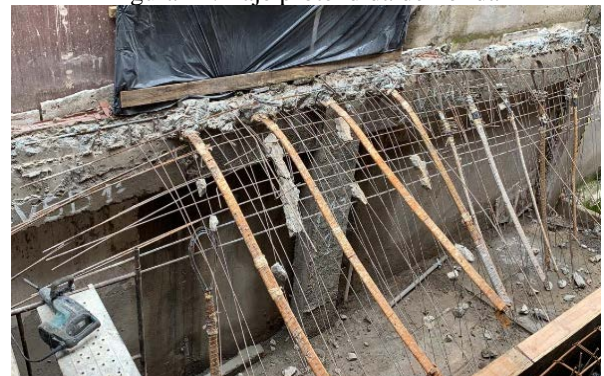
Figura 24: Laje protendida demolida
